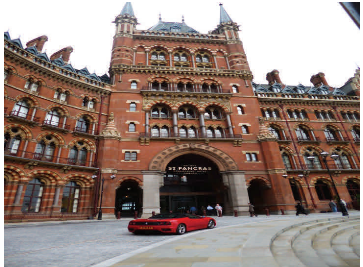
Figure3 St. Pancras Hotel, London, UK
